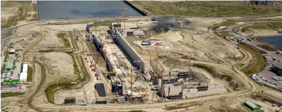
Figure 13. Construction of Kieldrechtsluis in Antwerp by means of a dry construction method.
