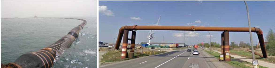
Figure 11. Floating pipe line and bridge construction of land lines over a road.
